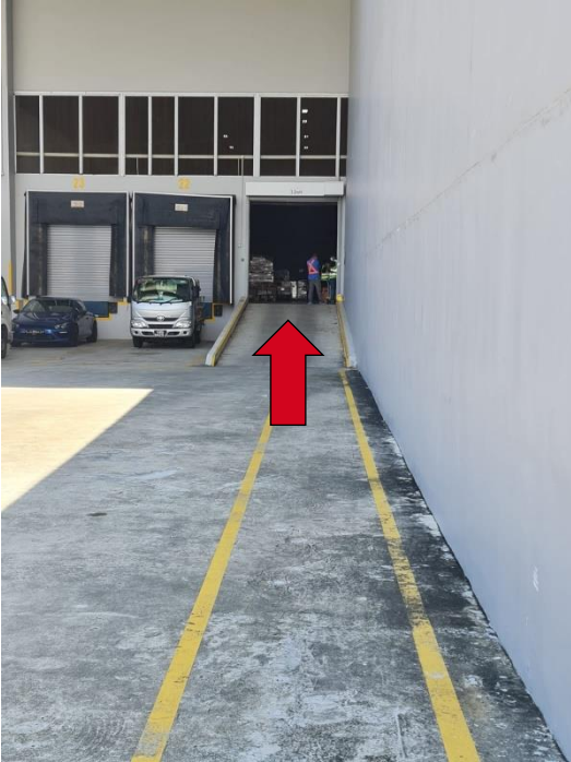
Bay 22 at Level 3
