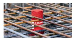
"Hilti cast-in devices create the opening for the pipes to go through and at the same time offer an integrated firestopping system. This product is so efficient and easy to install. We have installed 5,000 pieces and we had zero failures."
