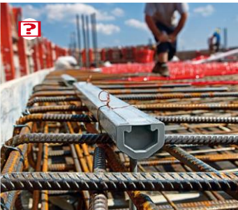
Cast-in anchors
