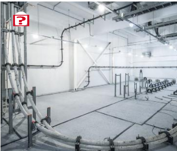
High voltage cabling supports
