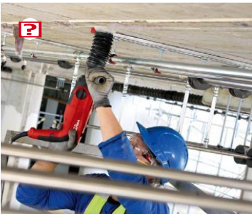
Post installed anchors
