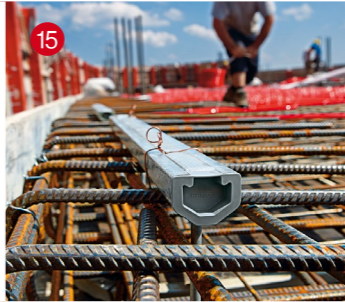
Cast-in anchors
